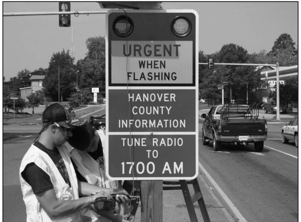
Using grant money and private sources, Hanover County has created a low-power AM radio system designed primarily to get out emergency messages. If you drive past one of these signs and the orange lights are flashing, that means an emergency message is being broadcast and please turn to AM 1700 (or call 365-1700 if you can't get the signal.) The newest sign was installed last month in Ashland and resulted from a donation by NextEra Energy Resources. Doing the work are Jonathan C. Passmore and D.J. Doane of Keeton Electrical.
